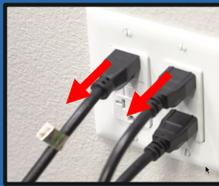
Unplug the electrical cords from the electrical outlet that includes the fountain dispenser and carbonator pump
