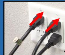
Plug in the electrical cords from the electrical outlet that includes the fountain dispenser and carbonator pump, turn co2 supply on. Remove all Bag-in-Box with expired date codes and dispose of properly.
